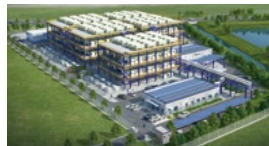
Bird's-eye View of Daesan Hydrogen Fuel Cell Power Plant
