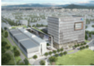
Aerial view of DRC in Gunpo
